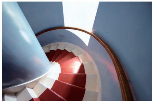
Photograph 2: Mull of Galloway Stairs
