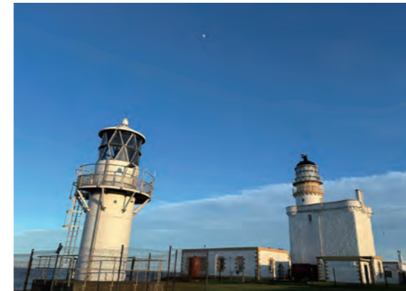
Photograph 1 : Historic Kinnaird Head Castle and Lighthouse alongside the modern NLB lighthouse
